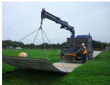
Trackway Installation
